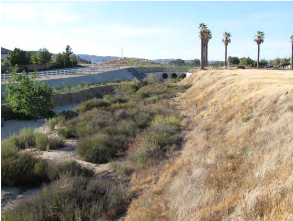
11) Stormwater drainage channel looking north.
