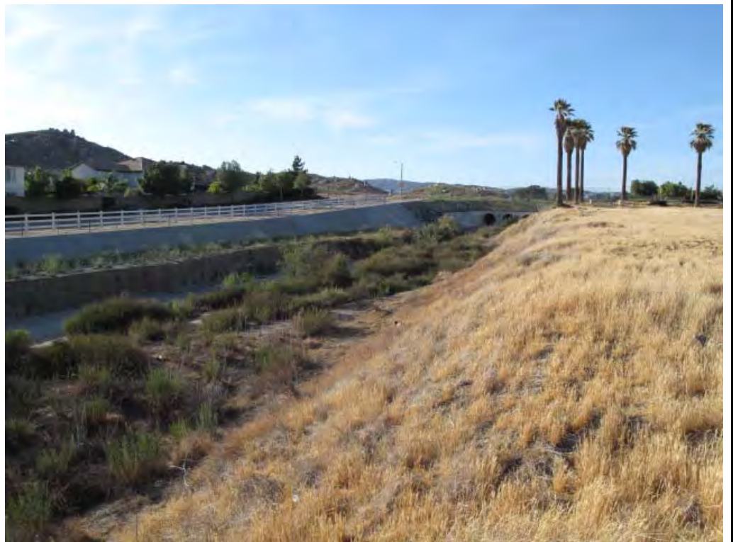
8) Drainage channel looking north.
