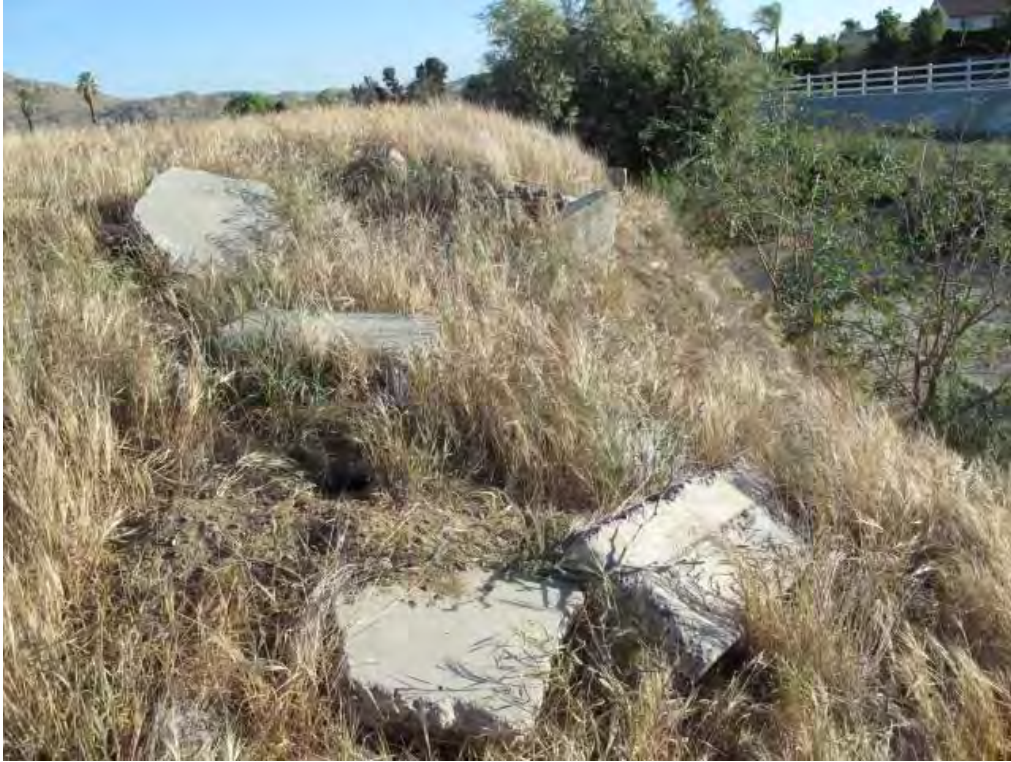
13) Remnants of concrete structures near drainage channel.
