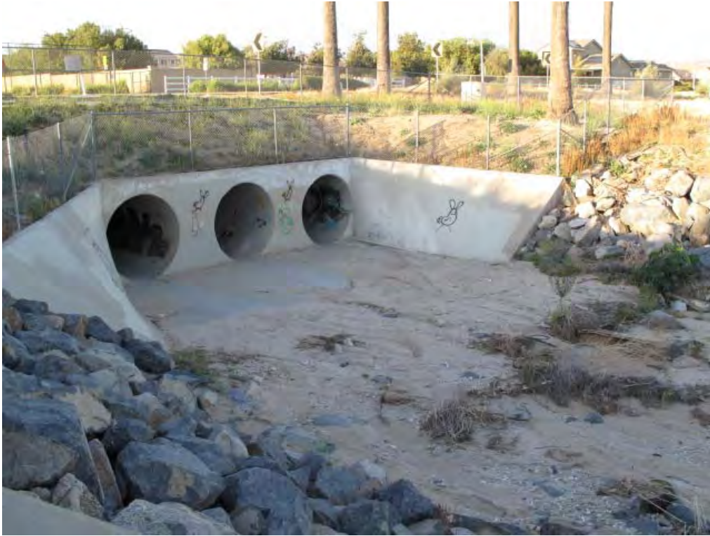
7) Concrete drainage culvert at adjacent stormwater channel.
