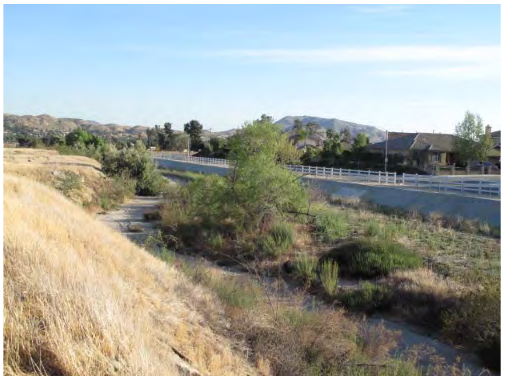
12) Stormwater drainage channel looking south.
